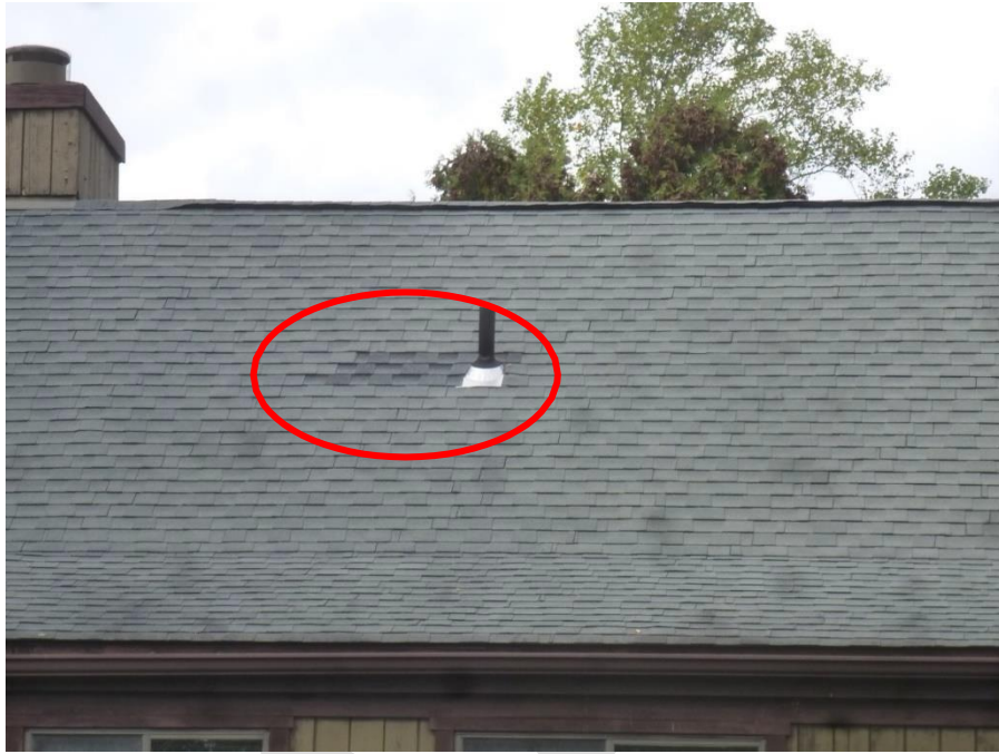
Photograph 11 Note patch at plumbing vent.
