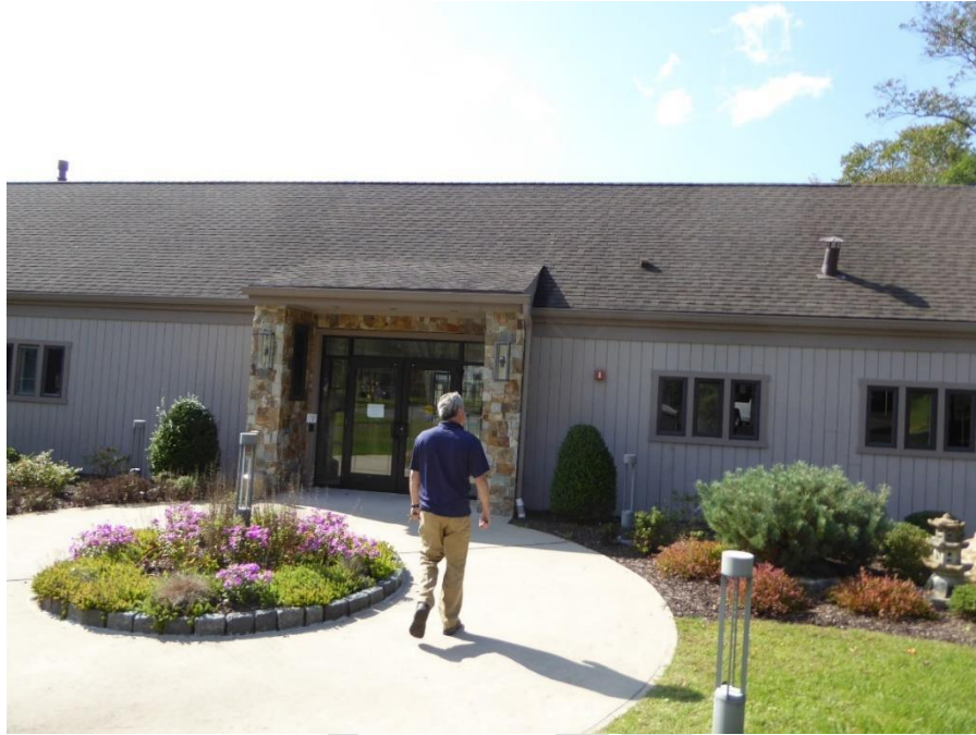
Photograph 1 Front Roof – North Club House
